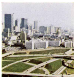
A highway system serving the distribution center of the Southeast.
